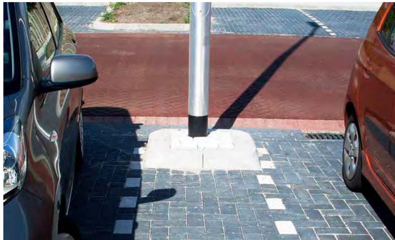
Lichtmast in parkeervak
